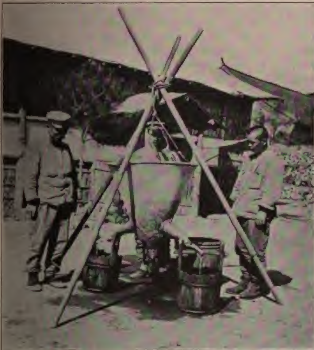
FIG. 61.—The Japanese field filter. ( Eshitzi filter. )
